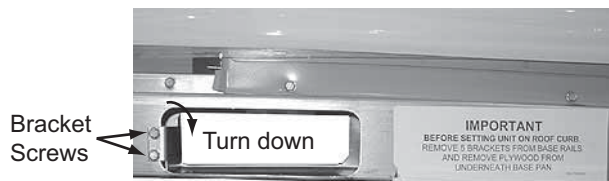
Figure 1: Unit Shipping Bracket
